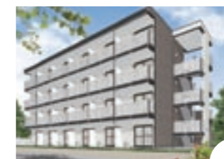
VILLA SUPERIO Introduced in 2006 Urban-style four-story structure targeting areas with high occupancy rates.
