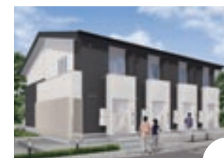
LEO GRANDIR Introduced in 2007 Family-type units in maisonette style equipped with a loft that makes use of space under the roof.
