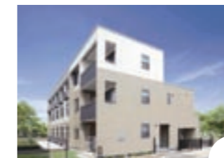
Lavo cerna Introduced in 2008 Partial leased residence that ensures the independence of the leased portion and the owner's residential portion.
