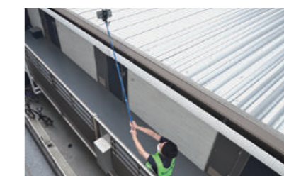
Building inspection in progress
